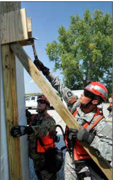
Practicing Their Skills: Members of the Missouri National Guard Homeland Response Force practice shoring up a concrete wall before conducting a search for injured people, Aug. 28, at the Mead Training Site.
