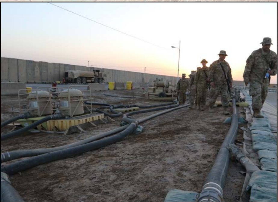
< Inspectors general from the 1st Theater Sustainment Command-Operational Command Post and petroleum specialists from Task Force Phoenix walk the fuel lines at a forward operation base in central Iraq to inspect the operations, recently. The 1st TSC is responsible for overseeing fuel logistics in multiple countries throughout Southwest Asia. (U.S. Army Photo by Sgt. Brandon Hubbard, 204th Public Affairs Detachment)
