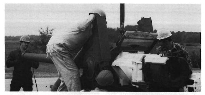
Aberdeen technicians mount a 105-mm gun on a test rig prior to proof firing. Elaborate measurements taken
