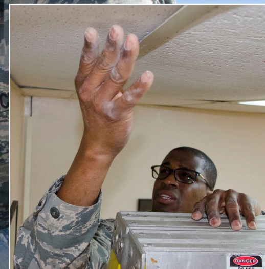
Above: Airman 1st Class Marchelle Charles places a new ceiling tile, at Joint Base McGuire-Dix-Lakehurst, N.J., April 19, 2017. Charles fixed a leak caused from winter weather that damaged ceiling tiles.
