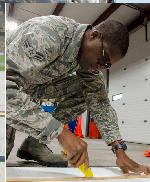
Above: Airman 1st Class Marchelle Charles places a new ceiling tile, at Joint Base McGuire-Dix-Lakehurst, N.J., April 19, 2017. Charles fixed a leak caused from winter weather that damaged ceiling tiles.
