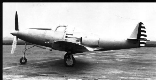
The prototype Bell XP-39 first flew in May 1939; for reasons, probably political and financial, the turbo-supercharger that can be seen mounted on the fuselage side, was deleted from production aircraft with a resulting drop in performance and ruining its future with the Army Air Corps. (public domain photo via Wikipedia)
