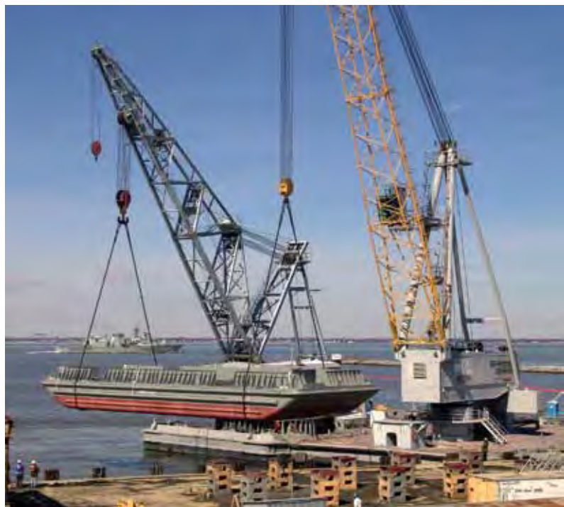
Opposite page and above photos: Crane and barge operations in Norfolk, Va.
