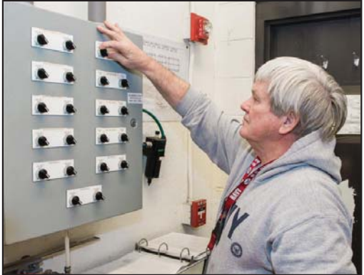
Clockwise: Edward Pitcavage, finish inspector, makes sure nozzles are the correct distance from a shelter before it starts to rain in the depot's rain test facility (top right), which is used to check the water tightness of equipment repaired or overhauled here. Right, Pitcavage confirms specific nozzles are selected according to customer requirements. Pitcavage works in the Continuous Process Improvement Directorate's Quality Control Division.
