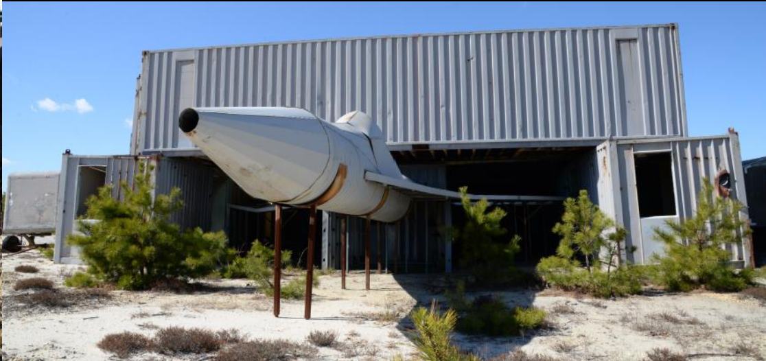
Below: A sheet metal fabricated aircraft shape is parked under a simulated hangar made of storage containers at the 177th Fighter Wing Det. 1 - Warren Grove Bombing Range in Ocean County, N.J. on Mar. 2, 2017. The storage containers, also known as Conex boxes, were acquired from the Defense Logistics Agency through the Reutilization Transfer Donation program.
