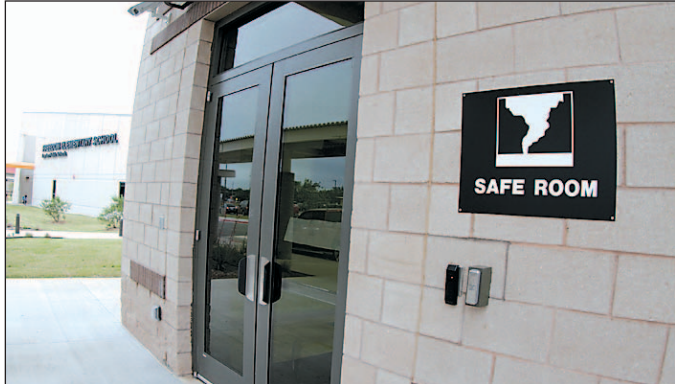
One of the safe rooms at Fort Sill's Freedom Elementary. Each safe room is built to FEMA standards designed to protect against an EF5 tornado.
