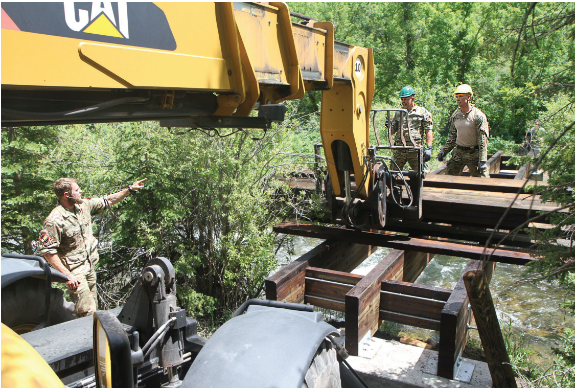
Danish 3rd Battalion Engineer Corps Soldier Sgt. 1st Class Jesper Tandrup (left), gives direction to Lance Cpl. Bo Andreasen (middle) and Lance Cpl. Abel Frederikson (right) while they remove cross beams from a bridge at Spearfish Falls in Spearfish Canyon, S.D., June 14. (U.S. Army National Guard photo by Spc. Joshua Quandt)
