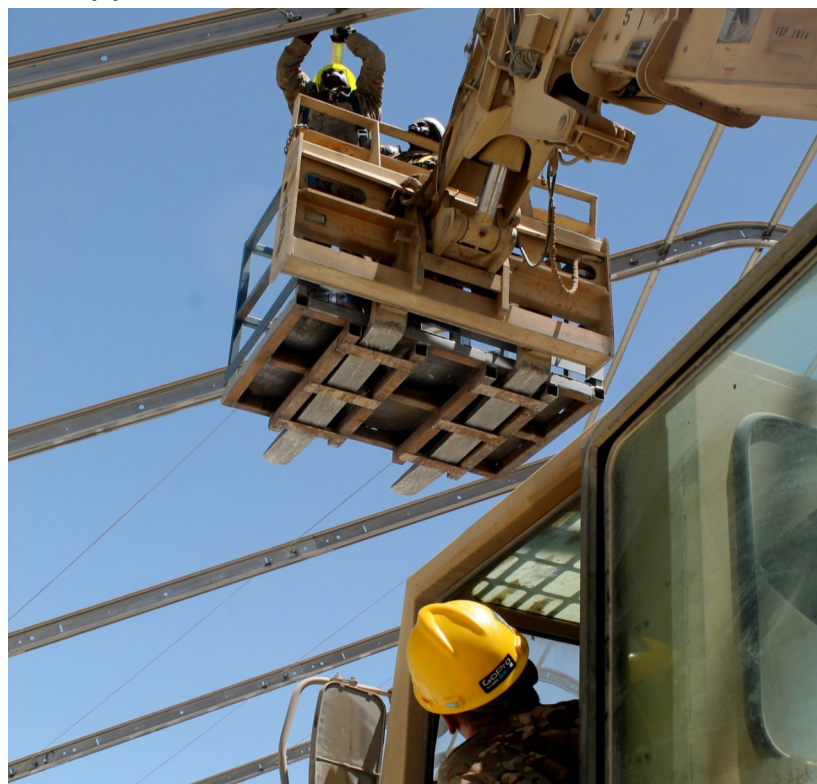
2 D Engineer Brigade Task Force Trailblazer Soldiers disassembling a Tension Fabric Structure in Afghanistan. (U.S. Army photo)
