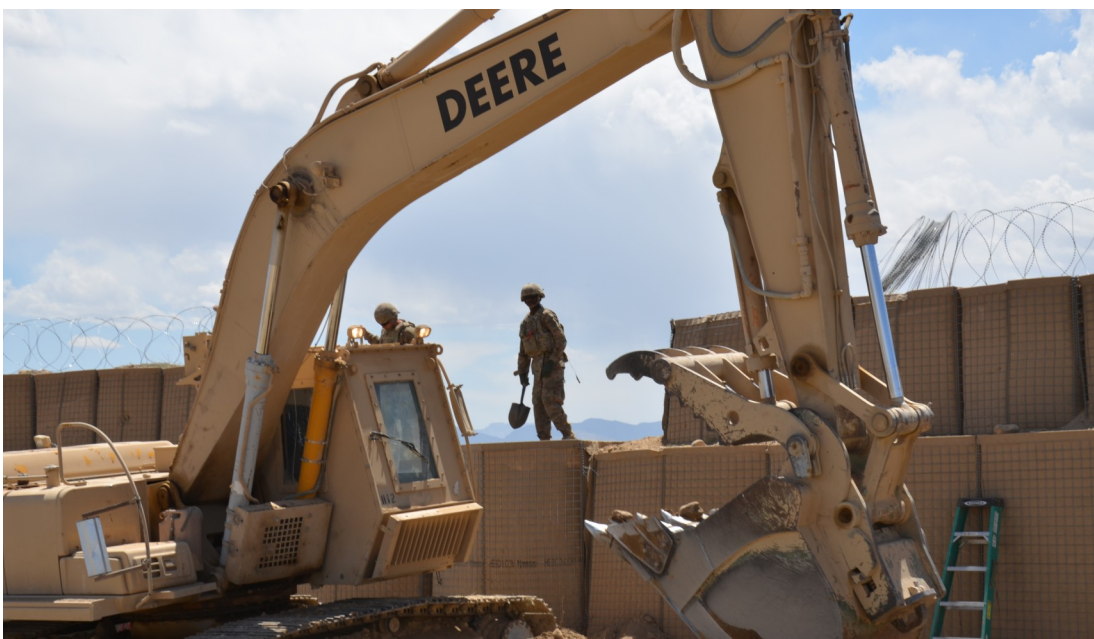
2 D Engineer Brigade Task Force Trailblazer Soldiers building a HESCO barrier in Afghanistan. As base footprints collapsed to "right-size" for Resolute Support it was often necessary to construct new force protection measures to ensure the safety of American forces and our allies. (U.S. Army photo by Capt. Drew Baughman)
