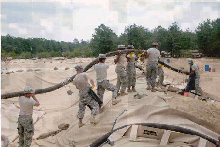
Army Reserve Soldiers with the 233rd Quartermaster Company out of Scranton Pennsylvania, carry a fuel pipe to set up a new 20,000 Gal. fuel bag as part of the Quartermaster Liquid Logistic Exercise (QLLEX) portion of the Combat Sustainment Training Exercise (CSTX) Global Lightning 2015 at Joint Base McGuire-Dix-Lakehurst, June 12, 2015
