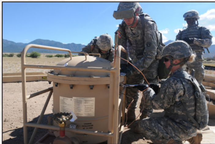
(Above) Army Reserve Sgt. Ryan Giegling inspect the filters in the filter separator tank during the Quartermaster Liquid Logistics Exercise (QLLEX) on Fort Huachuca, Ariz., June 10, 2015. According to Sgt. Vanessa Lauterwasser, clean rubber gloves must be worn while touching the filters to prevent any contamination in the fuel. Both Giegling and Lauterwasser are petroleum supply specialists assigned to the 383rd Quartermaster Company from St. Charles, Mo.
