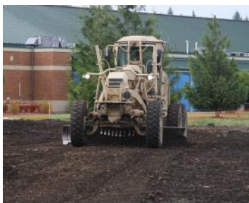
610th ESC Soldier uses a grader to level the new parking lot.
