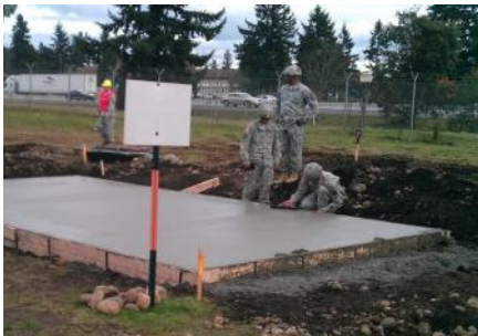
Final touches are put on the concrete pad before letting it set to dry.
