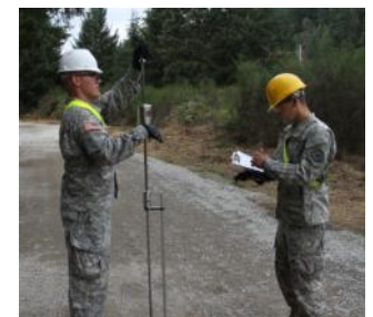
864th Soldiers test the compaction of the road to ensure it is ready for the next step.
