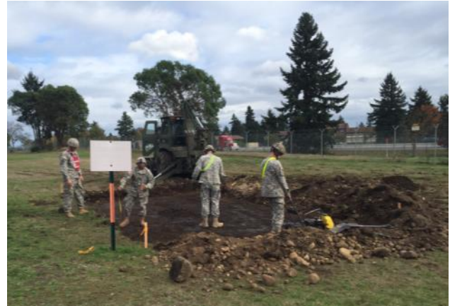
Soldiers with the 864th Engineer Battalion work on the foundation of what will be the concrete pad for the vehicle display.
