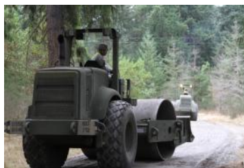
617th Soldiers compact the road to prepare for the asphalt.
