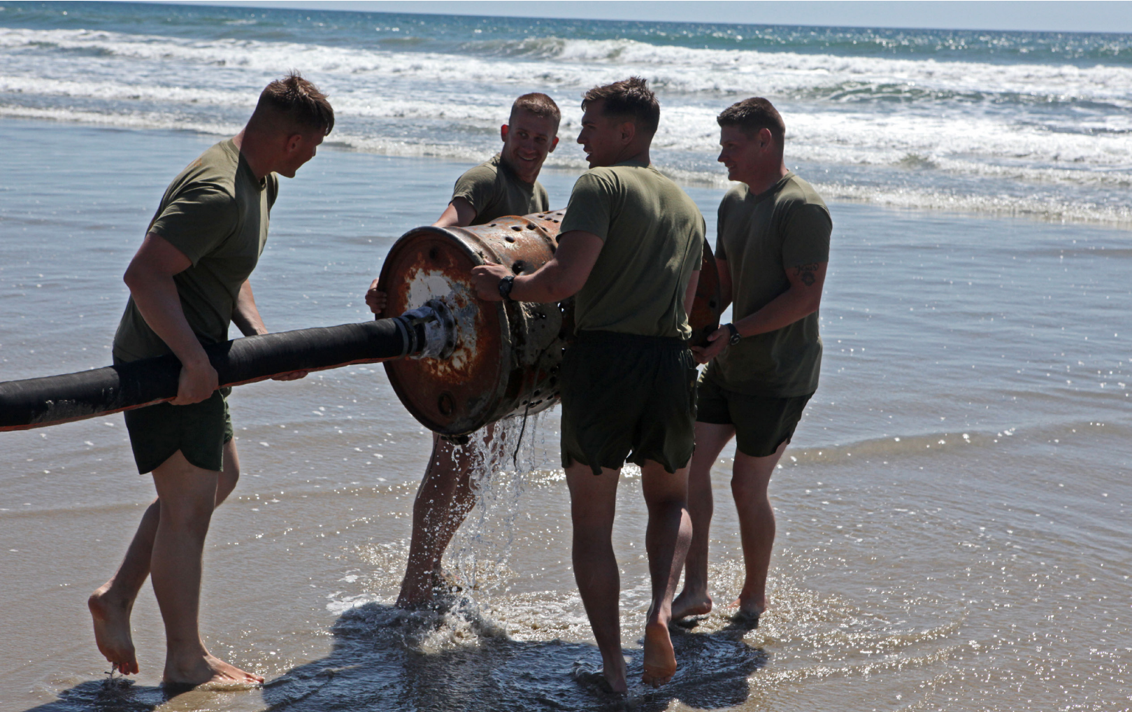
Marines with 2nd Platoon, Bulk Fuel Company, 7th Engineer Support Battalion, 1st Marine Logistics Group, practice inserting a basset pump into the ocean during a set-up of the Amphibious Assault Fuel System aboard Camp Pendleton, April 3, 2014. The AAFS allows for the receiving, storage, and distribution of 1.3-million gallons of fuel. This system uses a five-mile collapsible hose system to transport the fuel from a ship at sea to the units on shore. The basset pump would connect to the fuel hose from a ship at sea, and ensure that only fuel is in the hose before it reaches the pump onshore. The entire system consists of a vast layout of 33 fuel bladders, each holding 20,000 to 50,000 gallons of fuel.
