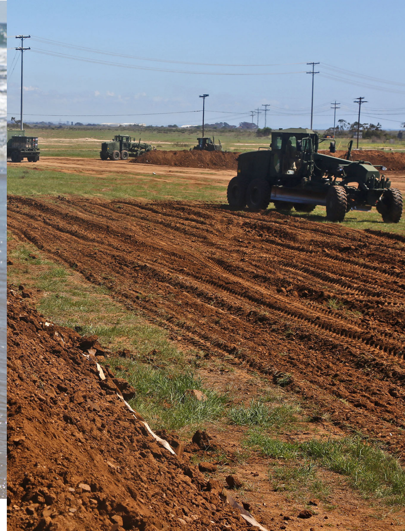
Left: Heavy equipment operators with Bulk Fuel Company, 7th Engineer Support Battalion, 1st Marine Logistics Group, build earth-berms in the early stages of constructing an Amphibious Assault Fuel System, Camp Pendleton, Calif., April 2, 2014. The AAFS allows for the receiving, storage, and distribution of 1.3-million gallons of fuel. The system consists of a vast layout of 33 fuel bladders, each holding 20,000 to 50,000 gallons of fuel, placed inside six-foot tall earth berms, as a safety measure, to contain any spillage should a bladder rupture.
