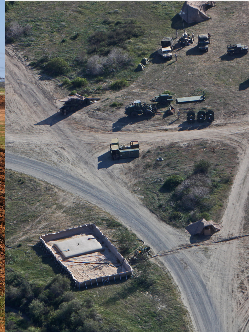
Left: Heavy equipment operators with Bulk Fuel Company, 7th Engineer Support Battalion, 1st Marine Logistics Group, build earth-berms in the early stages of constructing an Amphibious Assault Fuel System, Camp Pendleton, Calif., April 2, 2014. The AAFS allows for the receiving, storage, and distribution of 1.3-million gallons of fuel. The system consists of a vast layout of 33 fuel bladders, each holding 20,000 to 50,000 gallons of fuel, placed inside six-foot tall earth berms, as a safety measure, to contain any spillage should a bladder rupture.
