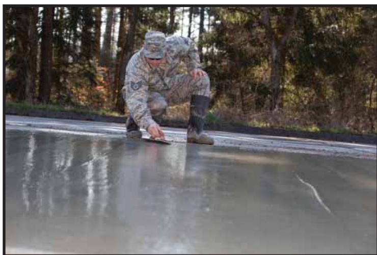
Staff Sgt. Steven Unglesbee, 175th Civil Engineer Squadron, Maryland Air National Guard, uses a float to prepare freshly poured concrete during the Silver Flag exercise, March 24, 2014, Ramstein Air Base, Germany. The Silver Flag exercise simulates training relevant to building and bed down of a bare base operation in a deployed environment.
