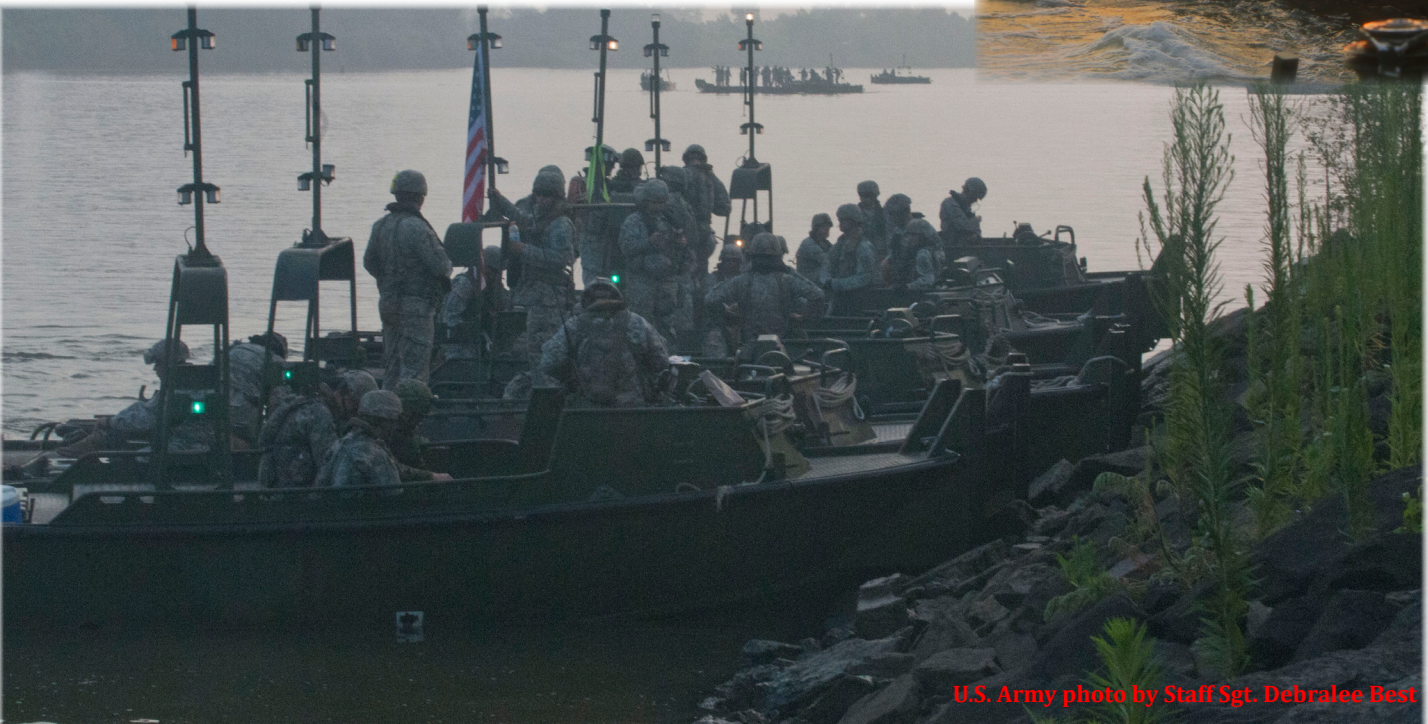
Below: Bridge erection boat crews await CH-47 Chinook helicopters to drop bridge bays into the Arkansas River.
