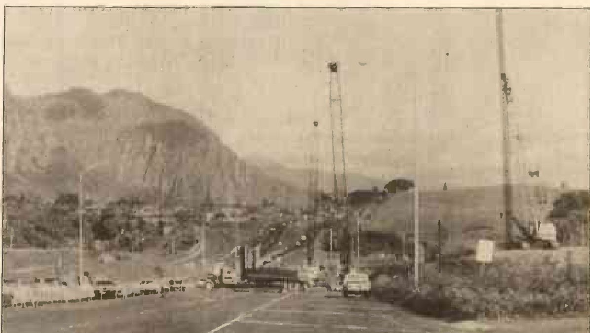
Pile-driving cranes block one lane of traffic on Kamehameha Highway to construct the overpass at the Halekou Interchange of the H-3.
