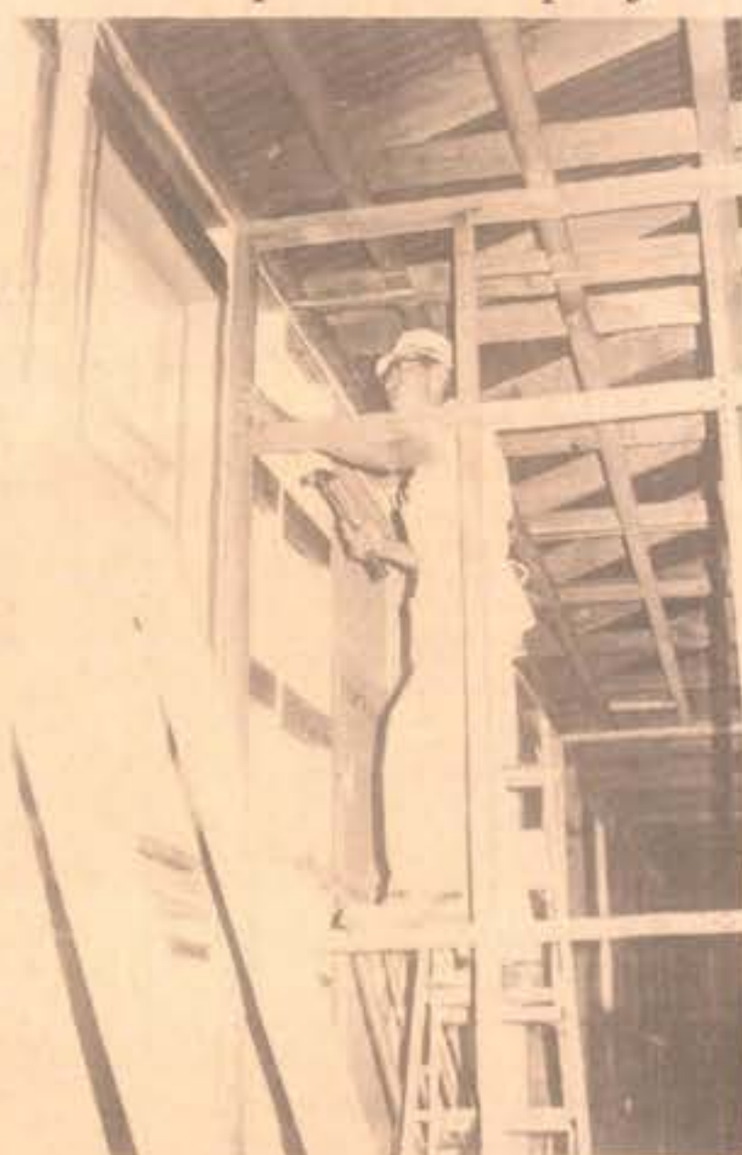
FRAMED — Clifford Kanehira of the Facilities Department secures the framework of a new wall at the station post office. The post office is being completely renovated to allow for more space and efficiency.
