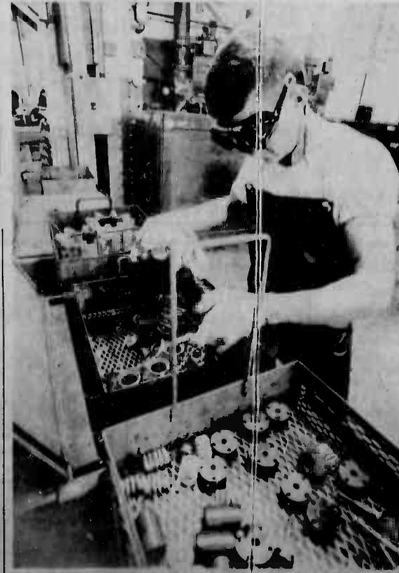
**BRAKE BATH** — Lance Corporal Ronald Mills, hydraulics mechanic, cleans the parts of an A-4 Skyhawk brake after the brake was disassembled. (Photo by Sgt Chris Taylor)
