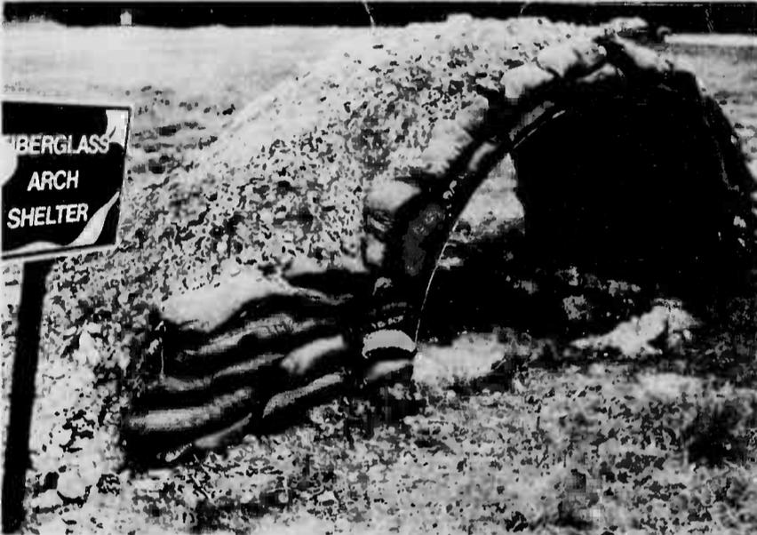
HOME SWEET HOME? — This protective shelter is being developed with the tank-killing TOW (tube-launched, optically-tracked, wire-guided missile) in mind. The shelter, plus 18 inches of dirt, allow the gun's crew to retaliate against enemy armor during bombardment. (Photo by Sgt Christopher Grey)
