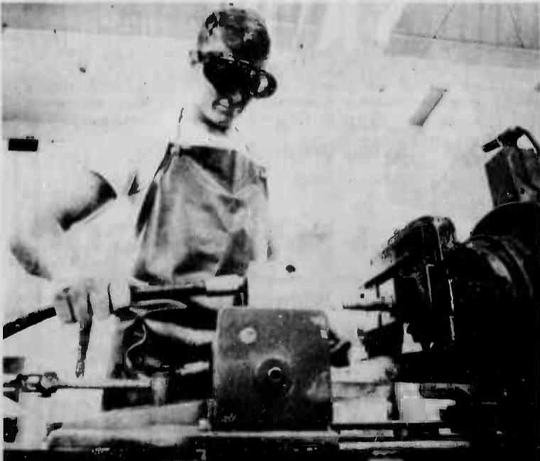
**HOSE MAKER** — Lance Corporal Ronald Mills, hydraulics mechanic, manufactures a hydraulic hose using the hose assembly
