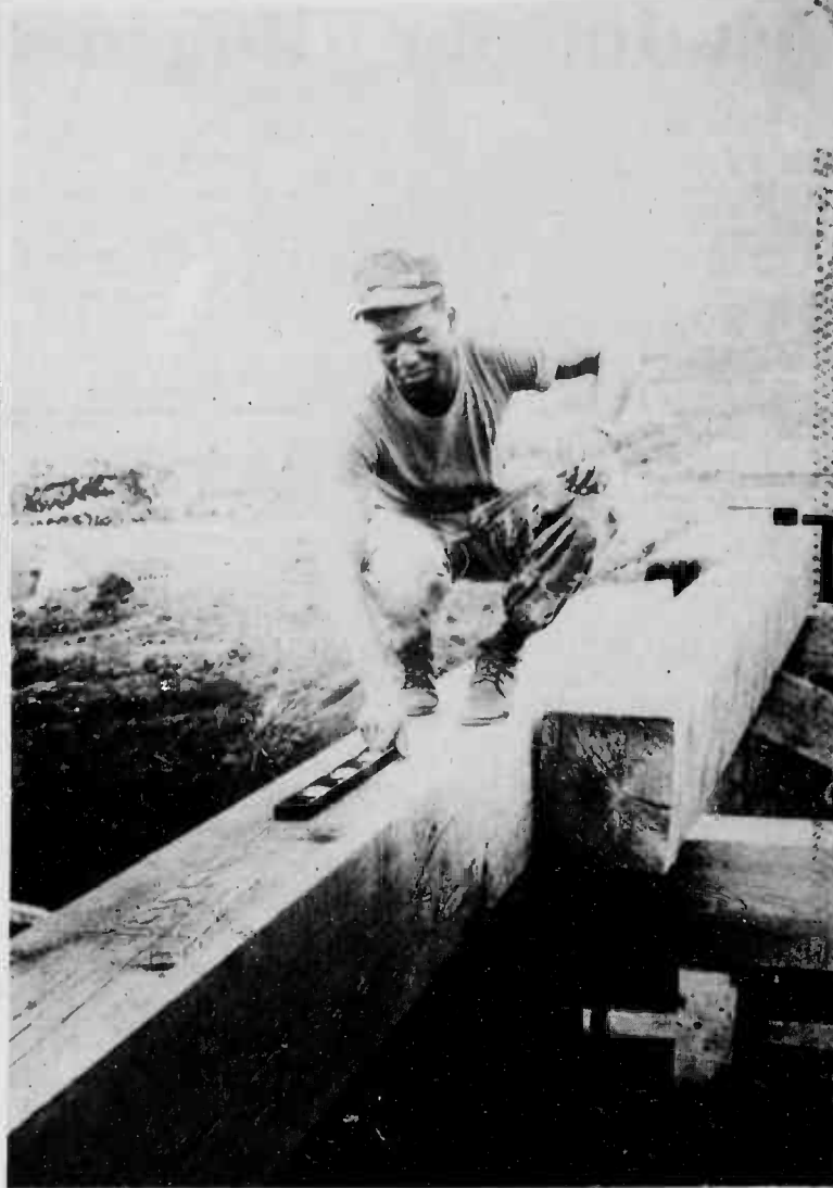
ON THE LEVEL — Lance Corporal Dennis Bowman checks the balance of a bridge support. LCpl Bowman's platoon recently took a giant training step by building a bridge.
