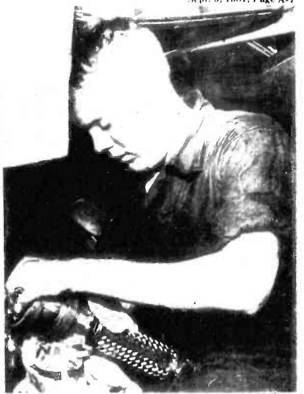
CLEANING UP - Lance Corporal Dan Geffe cleans the main fuel manifold of an F-4S fighter plane. LCpl Geffe is assigned to Marine Fighter Attack Squadron-235 and is part of the maintenance team that keeps the squadron's aircraft flying safely.
