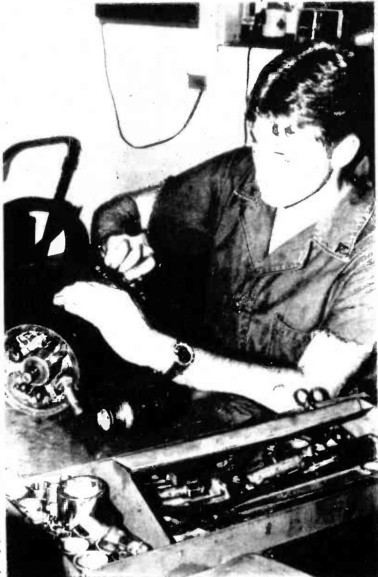
STARTING OVER — Lance Corporal Morrie Fink rebuilds a truck starter.
