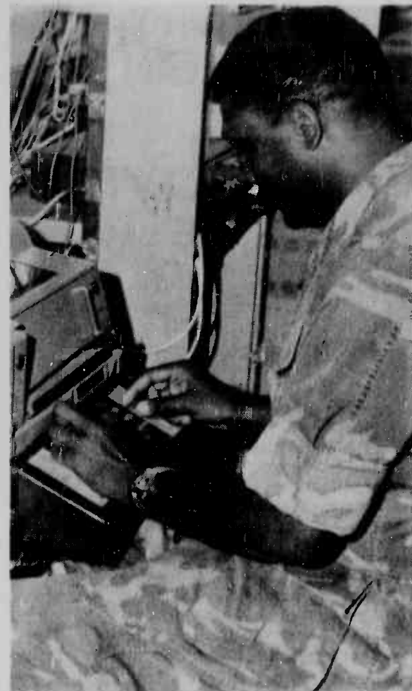
MESSAGE MACHINE — Staff Sergeant Hank Hugley, one of the two Marines of the K-Bay MARS station, types messages onto computer tape to be transmitted to other operators and eventually reach a serviceman, friend or family member. MARS-Grams are great morale builders.
