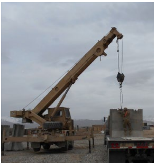
Spc. Michael Hatfield, a horizontal construction engineer for the 858th Engineer Company, attached to the 133rd Engineer Battalion, operates a 22-ton crane while Columbus, Miss. native, Spc. Michael Dement, also a horizontal construction engineer for the 858th, hooks and unhooks cable hooks to stage a concrete wall to be emplaced around a compound April 3. (U.S. Army photo by 2nd Lt. John Story,
