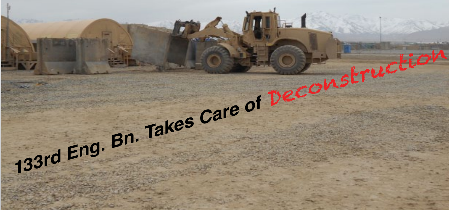
Ennis, Texas native, Pfc. Wesley Martin, a horizontal construction engineer for the Calhoun City, Miss.-based 858th Engineer Company, attached to the Portland, Maine-based 133rd Engineer Battalion, operates a 5-yard loader to emplace a barrier at Forward Operating Base Shank, Afghanistan April 3. (U.S. Army photo by 2nd Lt. John Story, 858th Engineer Company)
