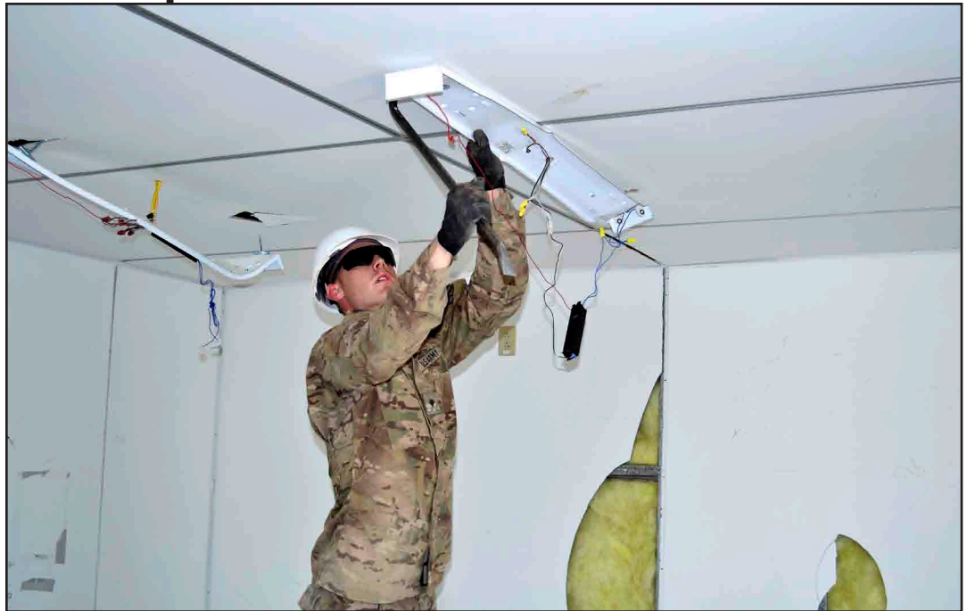
Ansonia, Conn. native, Spc. Mike Mobley, a carpentry/masonry specialist for the Marion, Va.-based 760th Engineer Company, attached to the Little Rock, Ark.-based 489th Engineer Battalion, uses a crowbar to take down a light fixture on a building that will be deconstructed during an engineer project March 29 at Camp Leatherneck, Afghanistan.
