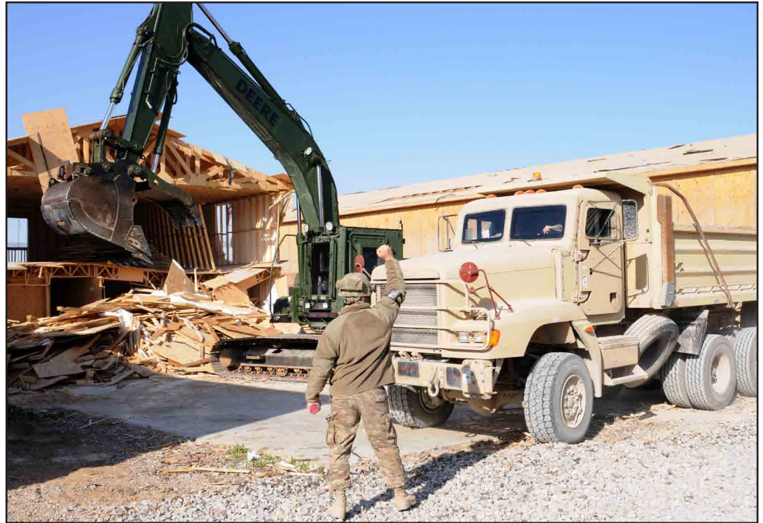
While deconstructing a building with a hydraulic excavator, engineers with the Little Rock, Ark.-based 489th Engineer Battalion pull up a dump truck to begin loading debris from the demolition Feb. 26 at Kandahar Airfield, Afghanistan.
