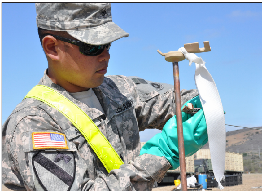
Sgt. Roland Amigo, petroleum supply sergeant with the 1017th Quartermaster Company out of Camp Pendleton, Calif., clamps a grounding wire to a grounding rod during a quartermaster liquid logistics exercise at Camp Pendleton.
