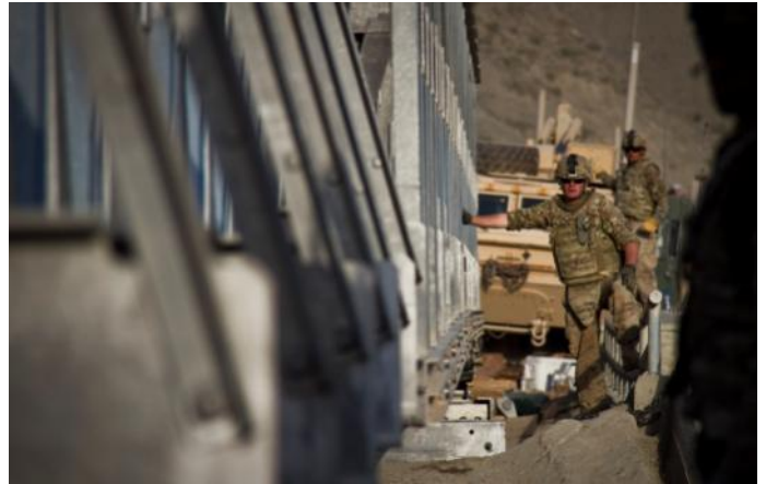
A Soldier from 1438th Multi-Role Bridge Co. monitors progress of a Mabey-Johnson bridge as it rolls across the gap it will cover.
