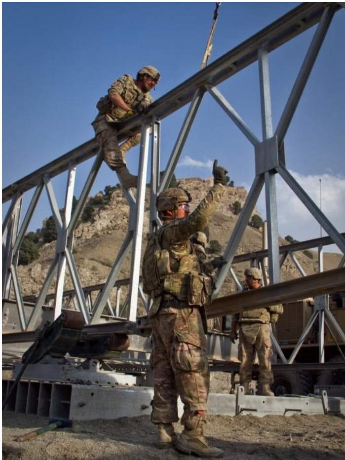
A Soldier signals to an excavator during construction of a Mabey-Johnson bridge in the village of Laka Tiza, Afghanistan, Sept. 2, 2013.
