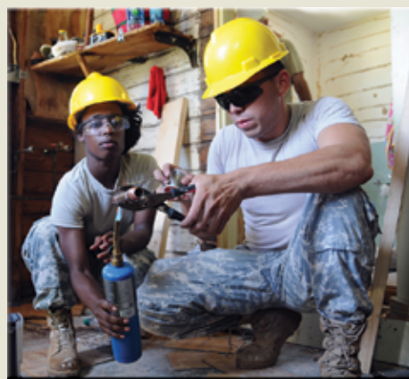
U.S. Army Pfc. Sherell Perry Webley, left, and Spc. Dennis Lopez, both carpentry masonry specialists, assigned to the 758 th Engineer Company, solder a copper pipe for the bathroom plumbing during the Innovative Readiness Training with Rebuilding Miami Together project in Perrine, Fla., June 10, 2013.
