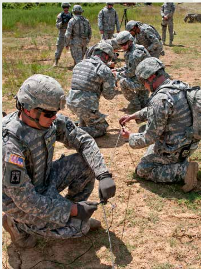
U.S. Soldiers assigned to the 854 th Engineer Battalion (Forward Support), connect their shaped charges to the main ignition line at the demolition range at Fort Chaffee, Ark., July 18, 2013. The shape charge will provide a proper size hole for the 40 pounds of cratering charge that will be placed in later.
