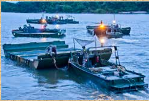
U.S. Army combat engineers with the 671 st Engineer Company (Multi-Role Bridge), 74 th Engineer Company (MRB) and 459 th Engineer Company (MRB), connect Mark II bridge erection boats to bridge sections on the Arkansas River during Operation River Assault at Fort Chaffee, Ark., July 24, 2013. The bridge sections were assembled together to form one fully functional bridge across the river. (U.S. Army photo by Sgt. Dalton Smith, 354 th Mobile Public Affairs Detachment)
