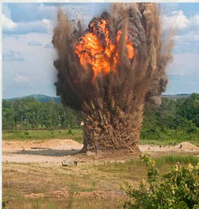
U.S. Soldiers detonate 170 pounds of high explosives during a demolition exercise at Fort Chaffee, Ark., July 18, 2013. Combat engineers use cratering charges to create defensive positions and other necessary emplacements.
