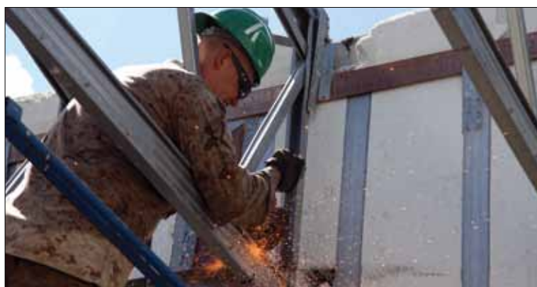
Lance Cpl. Jesse R. Gribble slices through a piece of metal Aug. 9 while deconstructing a dilapidated building on Camp Hansen. The building, along with another, presented a hazard to both personnel, as well as the equipment being stored in them due to deterioration from severe weather. Gribble is a combat engineer with 9th Engineer Support Battalion, 3rd Marine Logistics Group, III Marine Expeditionary Force.
