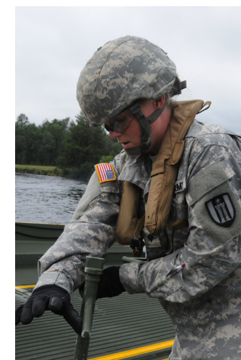
Spc. Alexic Cook, a bridge crewmember with the 739th Engineer Battalion, uses a T-rod to affix a floating bridge bay during the Combat Support Training Exercise 86-13-01 at Fort McCoy, Wis., in August. (Photo by Spc. Hector Corea, 366th MPAD)
