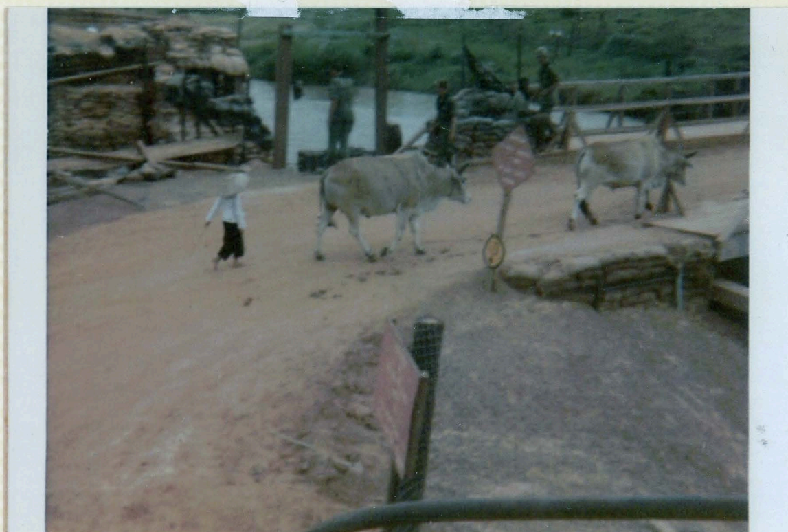
The Bridge at Dau Tieng
