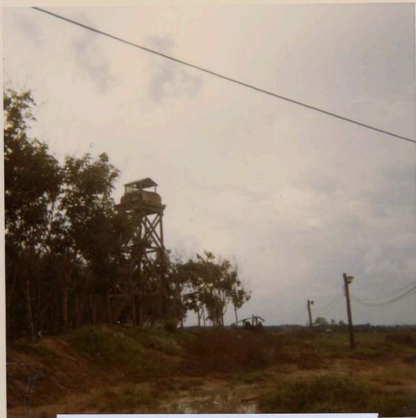
GUARD TOWER DAU TIENG
