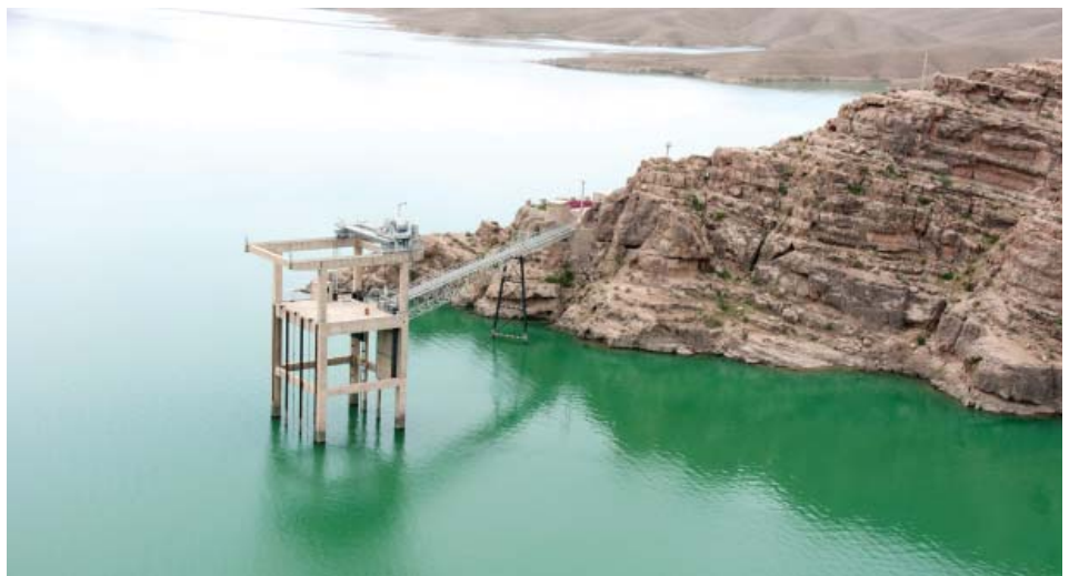
The Kajaki Dam intake structure is in need of rehabilitation. The U.S. Army Corps of Engineers awarded a contract in late January 2013 that will repair key components of the structure. (USACE Photo by Karla Marshall).
