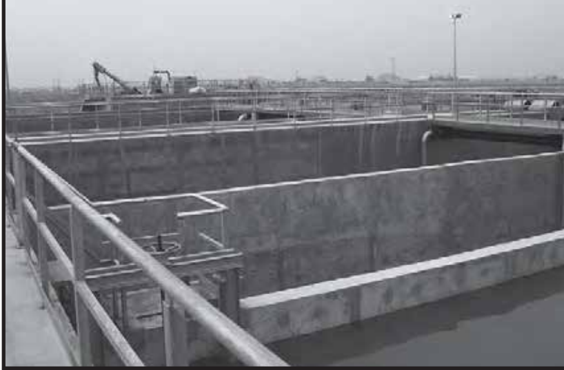
A new sewage treatment plant
