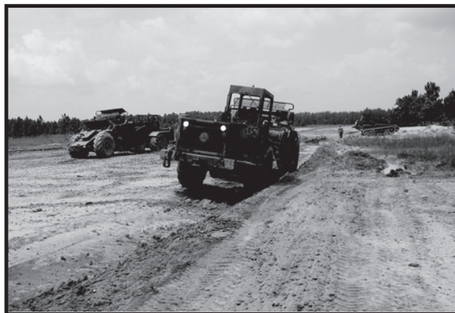
Grading, leveling, and drainage construction operations using the 613BS Scraper and DEUCE
