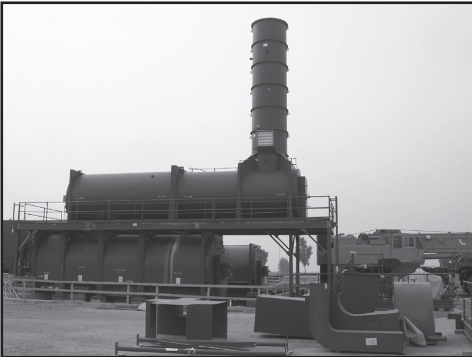
Constructing an incinerator
