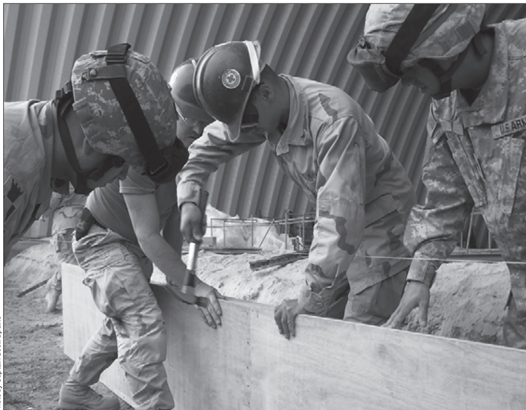
Seabees and Soldiers combine skills to erect formwork during a project.
