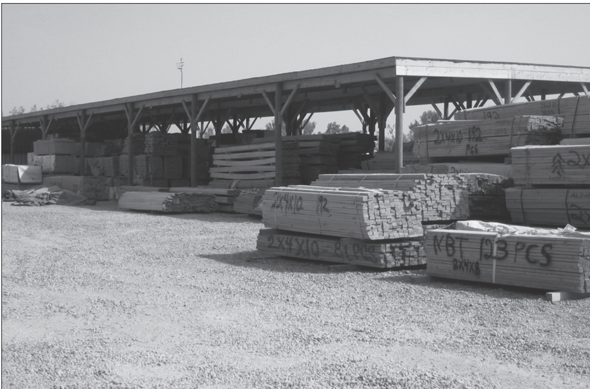
A pole barn—designed and built by the 130th Engineer Brigade—protects stocks of lumber, plywood, and cement from the elements.
