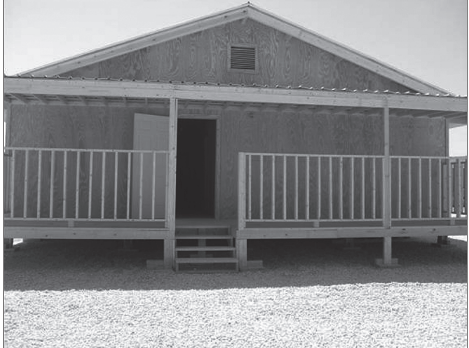
A SWA hut nears completion.
