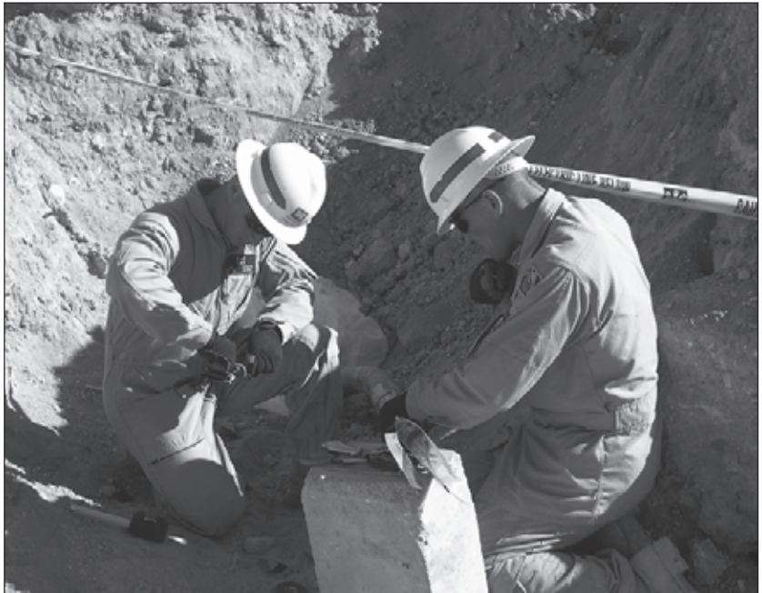
Soldiers splice a medium-voltage distribution cable.
