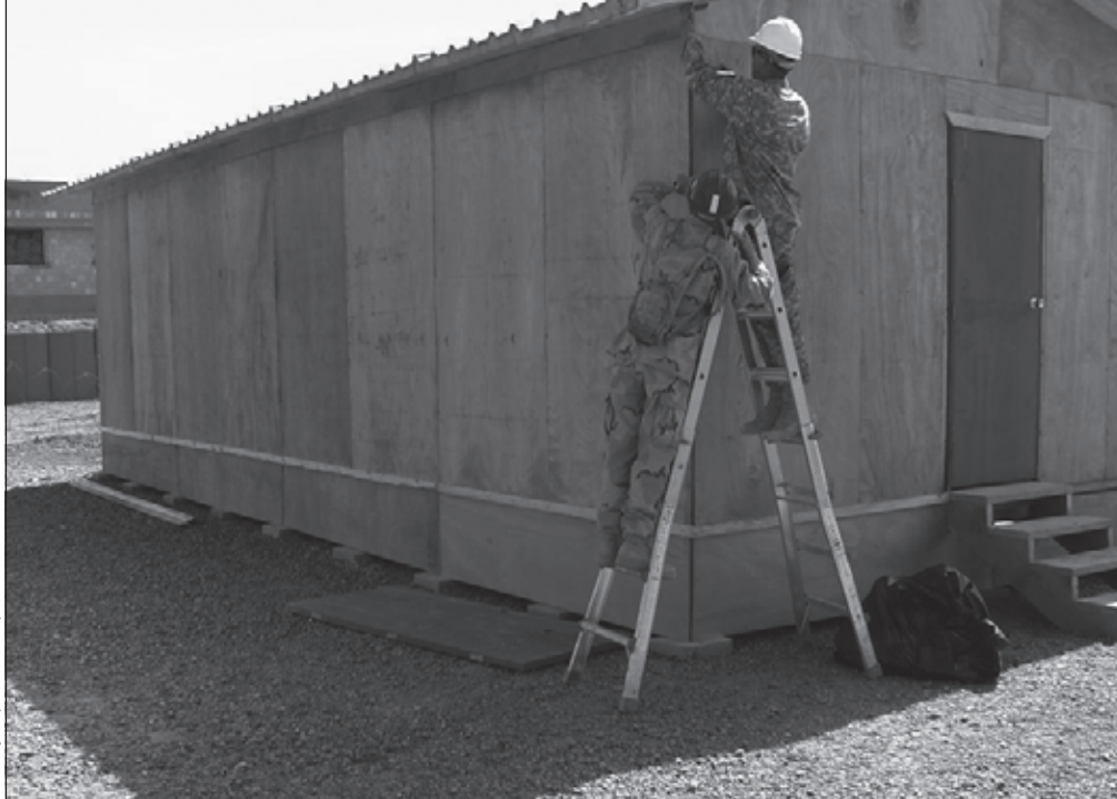
A Seabee and a Soldier work side by side hanging trim on a SWA hut.
