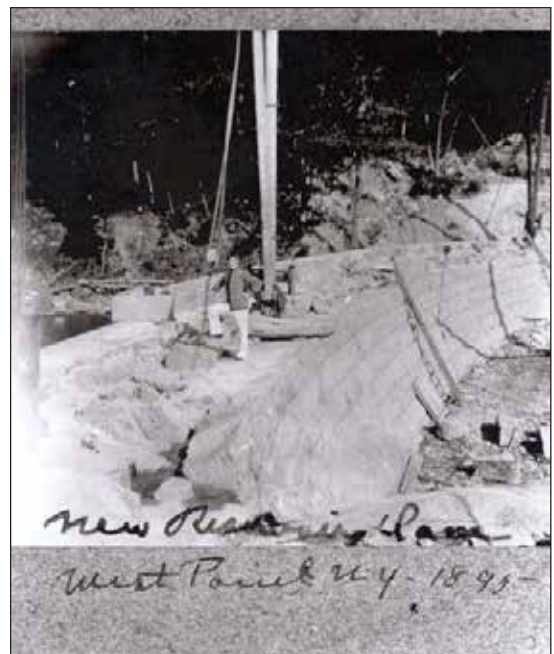
A Corps engineer stands on the recently constructed Lusk Reservoir Dam in 1895.
