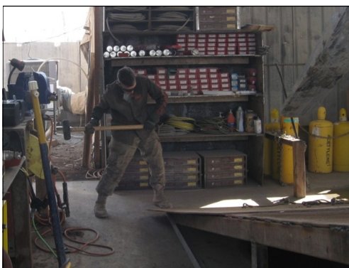
Kandahar- SPC Zachary Belisle uses a sledge hammer in conjunction with the 10K forklift to better align the plate steel used in emplacement of the ramps outer skin. The difficult alignment of the pieces was compounded by the weight of the steel along with the angle at which they had to be
