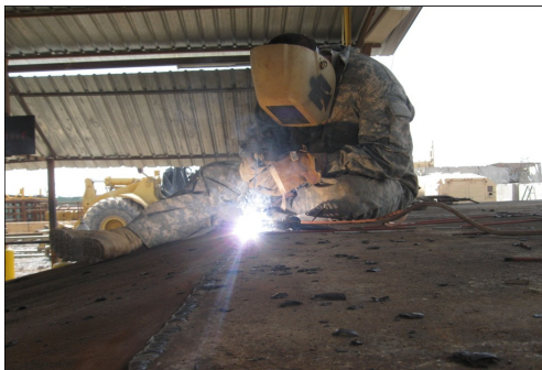
Kandahar- SPC Stephen Fadden welding the seam between the ramp and platform portions of the loading dock. The welding portion of the project was a critical piece in order to ensure the structural integrity of
