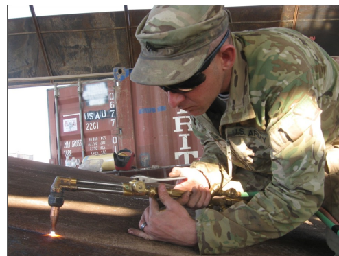
Kandahar- SGT Smokey Lyons uses a cutting torch to trim the dock plate of the ramp to facilitate a cleaner better fit to enable the
