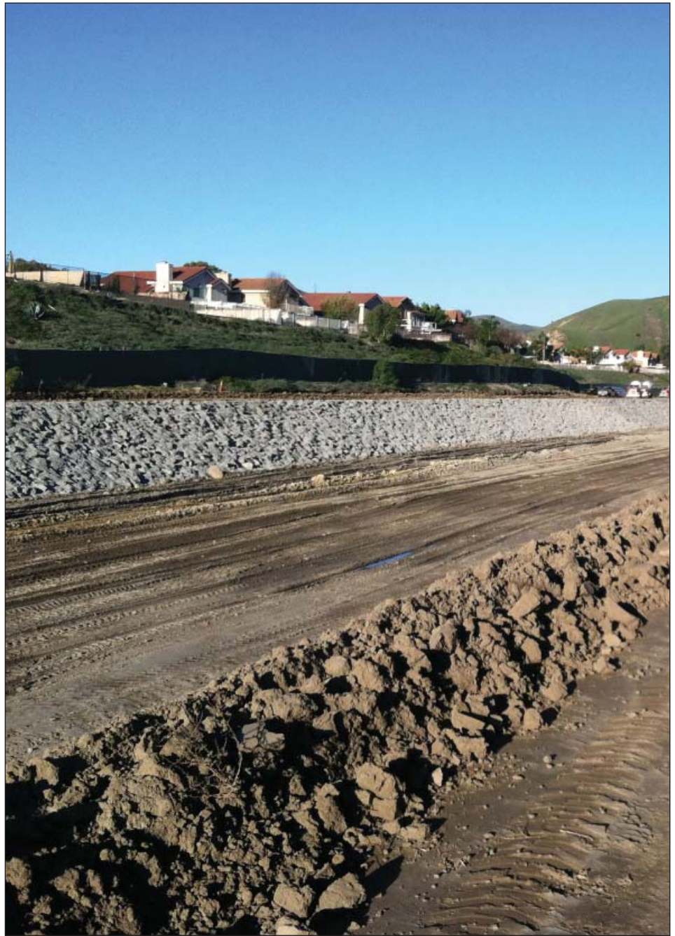
Grouted stone bank protection placement is part of Phase 2A of the Lower Santa Ana Bank Erosion Protection Project and is made of a two-foot-thick combination of stone and grout. (USACE photo by Chadi Wahby)
