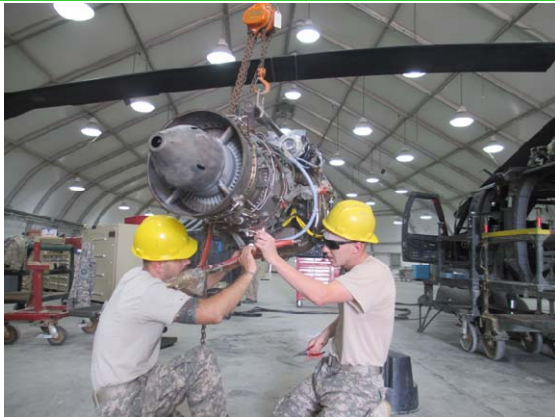
SPC Shaun Petersen (left) and SPC Russell Sternal (right) service and repair the powerplant (engine) of a UH-60 Blackhawk.
