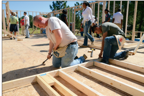
Spc. Christopher S. Leigh, 25 Q assigned to B Co., and Spc. Rudy L. Frias, a 25 Q assigned to C Co. 50th ESB, nail the framework of an inner wall together. This is part of a volunteer effort of nineteen Soldiers of the 50th ESB to construct and raise the walls of the future Thomas family home in Aberdeen, N.C., Oct. 16, 2012.
