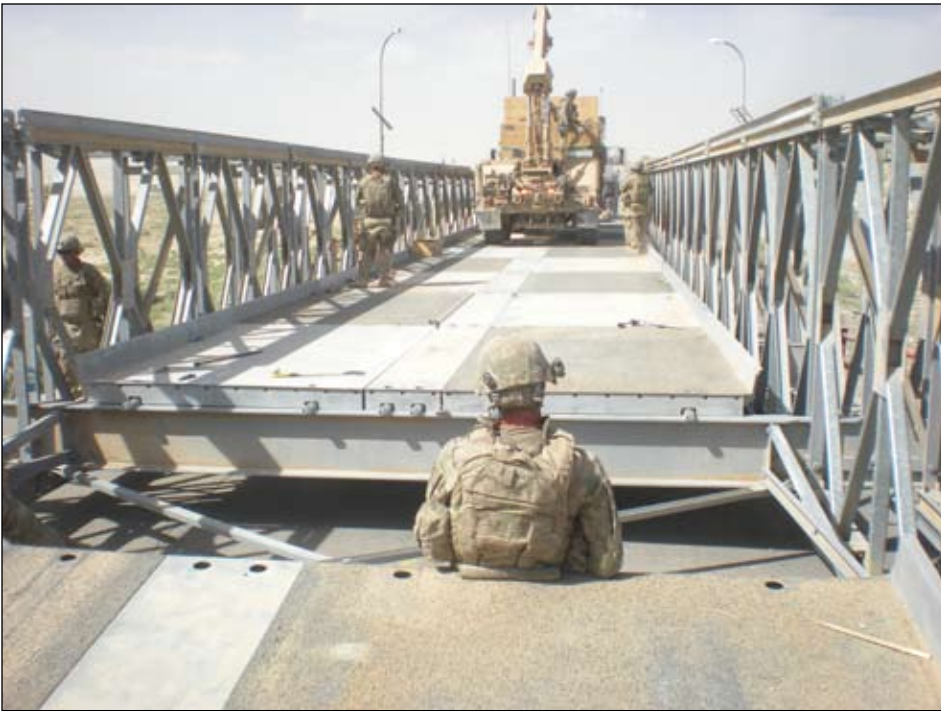
Photo by U.S. Army Sgt. 1st Class Jason Armano, Joint Task Force Empire Engineers of Joint Task Force Empire construct a bridge in southern Afghanistan. Bridging operations were a major concern for the JTF partnered with IJC assets throughout the country to maintain bridge crossings open for coalition and Afghan traffic.
