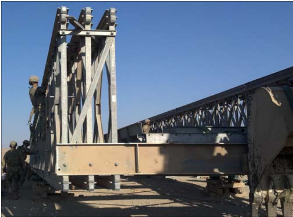
Photo courtesy of U.S. Army Col. John Elam, JTF Empire Military engineers emplace one of two 17-bay Acrow bridges during OGG. Members of JTF Empire, TF Warhammer and the 132nd Multirole Bridge Company (MRBC) installed the first Acrow bridge Nov. 22-24.
