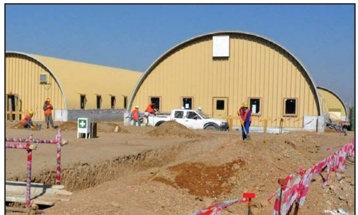
Photographed is an expansion project on Camp Zafar in Herat province. An Afghan-owned and operated company is constructing the facilities in compliance with globally-recognized standards.
