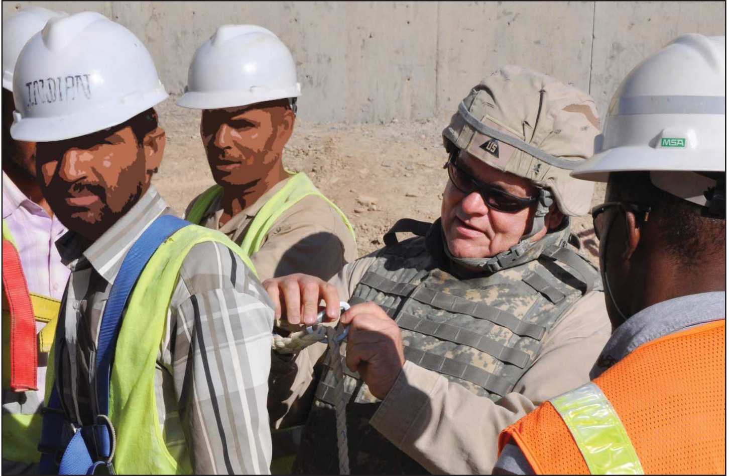
Jeff Ice, a safety and occupational health specialist who deployed to Kandahar from the USACE New York District inspects the harness on a construction worker at a job site. Construction is one of the most dangerous industries, not only in Afghanistan, but worldwide. As such, safety and occupational health specialists inspect job sites and equipment, and observe practices to ensure safety standards and regulations are followed. (Image has been altered to protect the identity of the laborers photographed.)
