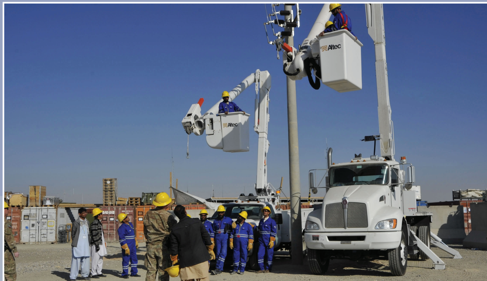
USACE's 249th Prime Power Battalion non-commissioned officers organized and conducted training that taught Afghan DABS engineers and technicians the fundamentals of safety, power line maintenance, operating "bucket trucks" that allow linemen to reach the top of utility poles, operating augur trucks used to drill and emplace utility poles.
