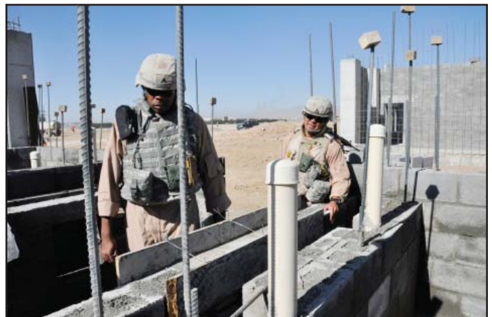
Ira Dorsett, a structural engineer, (left) and Benny Apuya, (right) a quality assurance and construction representative, both with the Afghanistan Engineer District-South inspect the masonry block work for a concrete sink at the Kandahar Regional Military Training Center construction site.
