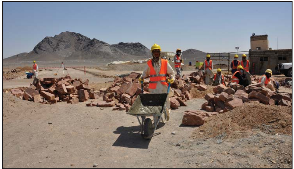
The U.S. Army Corps of Engineers is overseeing about 260 construction, operations and maintenance and service contracts in the south and west of Afghanistan. Construction contracts for project sites like this require close oversight and management. (USACE photo.)
