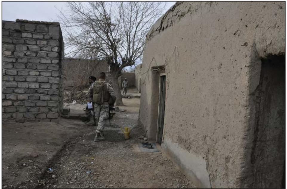
Before construction on a new police station in Tor Gundi, facilities were old, decrepit buildings and some shacks for cooking, sleeping and working as photographed above.
