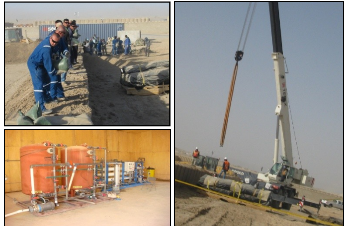
Clockwise from top left: Logistics Civil Augmentation Program performance contractor Fluor workers work on the Camp Marmal water point where they are completing work to support and expand water production. Also shown is part of the reverse osmosis equipment used to purify water. Water is brought to potable and disinfected non-potable standards for use on Camps Marmal and Pratt.
