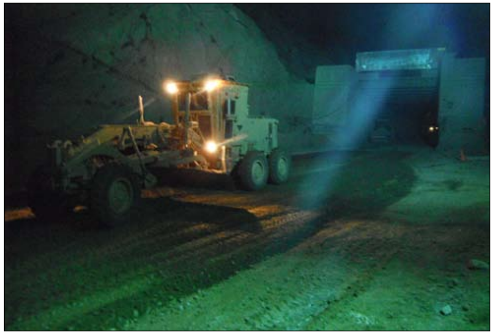
Photo courtesy of Operation Mountain Blade Personnel Soldiers work on improving the road surface of the Salang Pass during Operation Mountain Blade in Parwan Province, Afghanistan, recently. The engineers worked primarily at night due to the large amount of vehicles using the roadway every day.
