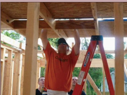
Staff Sgt. Foster uses his prior MOS skills (12B) to hang joists
