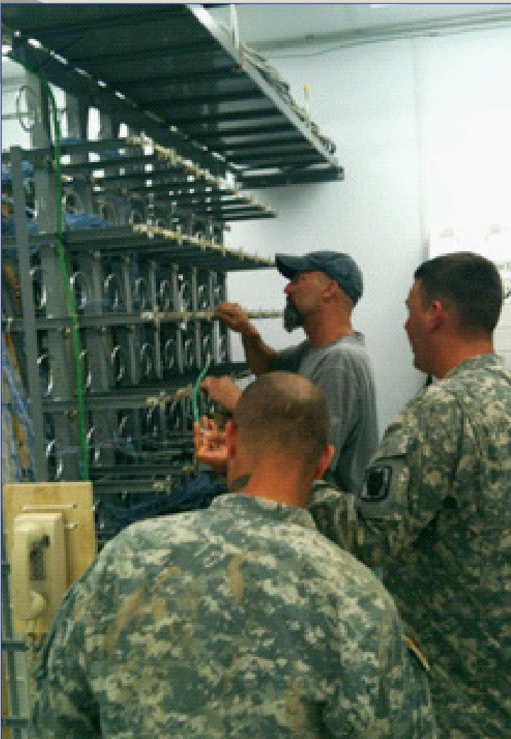
Sgt. Christian and Spc. Proctor prepare the 300-pair cable for installation.
