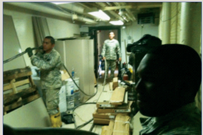
Sgt. Christian and Spc. Proctor prepare the 300-pair cable for installation.
