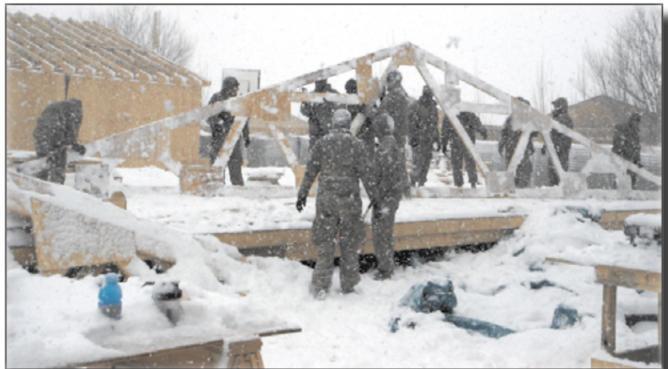
photo courtesy of Task Force Mad Dog Public Affairs Soldiers from the 236th Vertical Construction Company construct trusses at Forward Operating Base Warrior.
